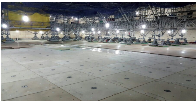
Erected KC-1 Insulation Panel
